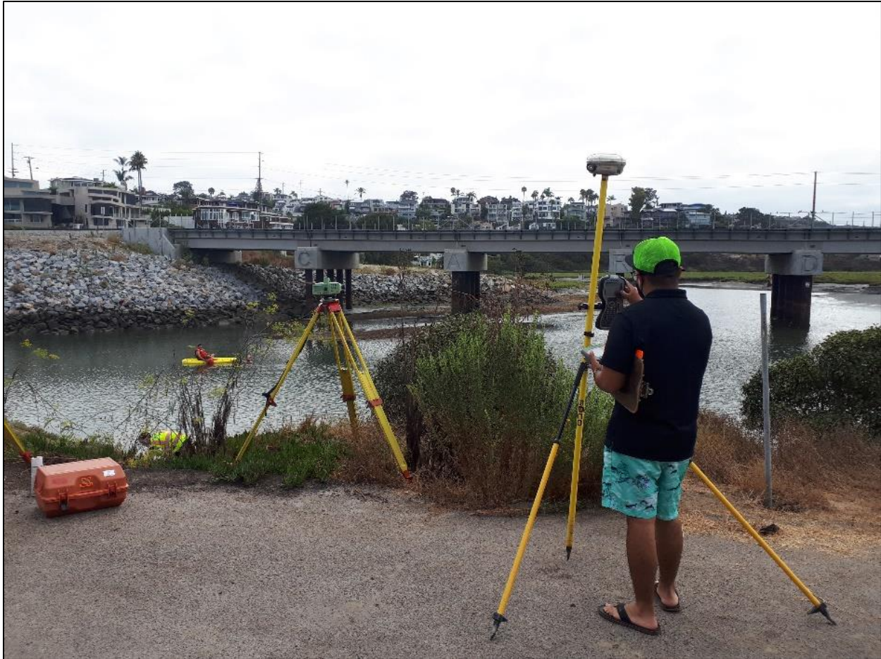
Figure 2-4: Water surface elevation survey near the Tidal Inlet Channel station.
